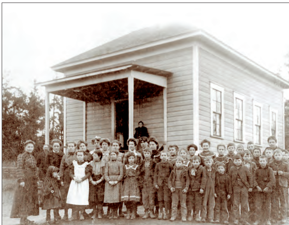
ABOVE: Esther Skarstedt Brown and her class pose in front of Glenwood School in 1902. The building still stands at Northeast 134th Street and 87th Avenue.
